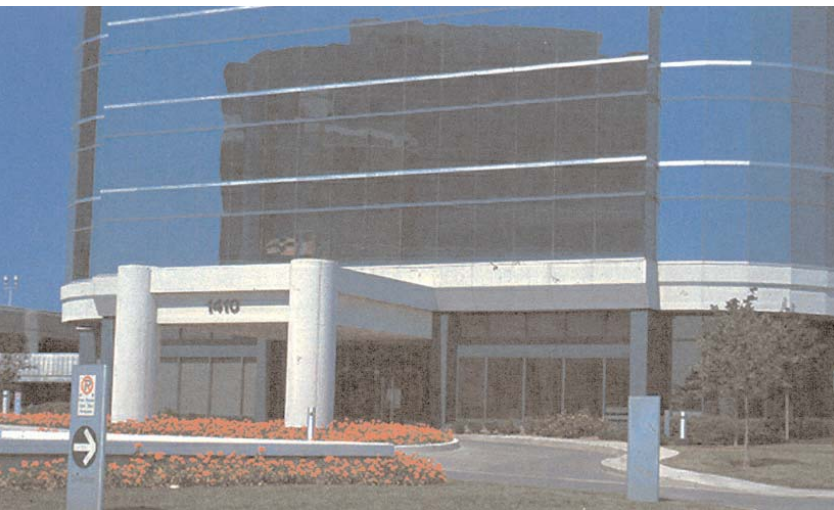
Fig. 6 – Structural Silicone Glazing System
