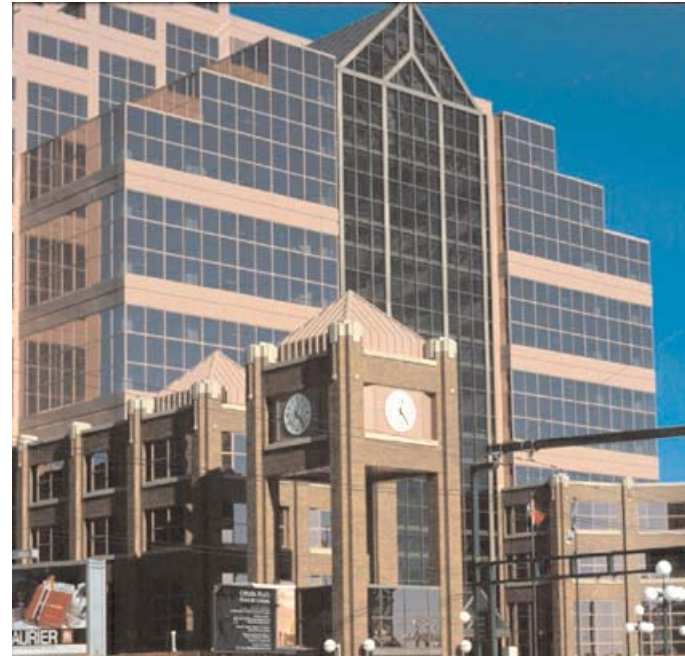
Fig. 1 Curtain Wall With Granite Spandrel Panels
