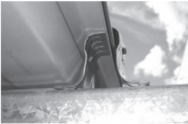
Figure 9.1.10b Position the 'S' clips over the male lapping rib of the cladding.
